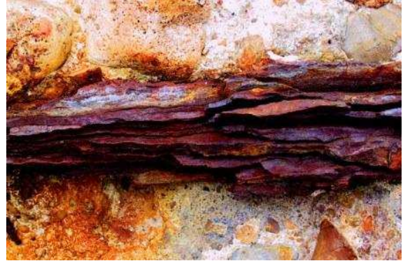
Figure 5: Rusty Rebar
